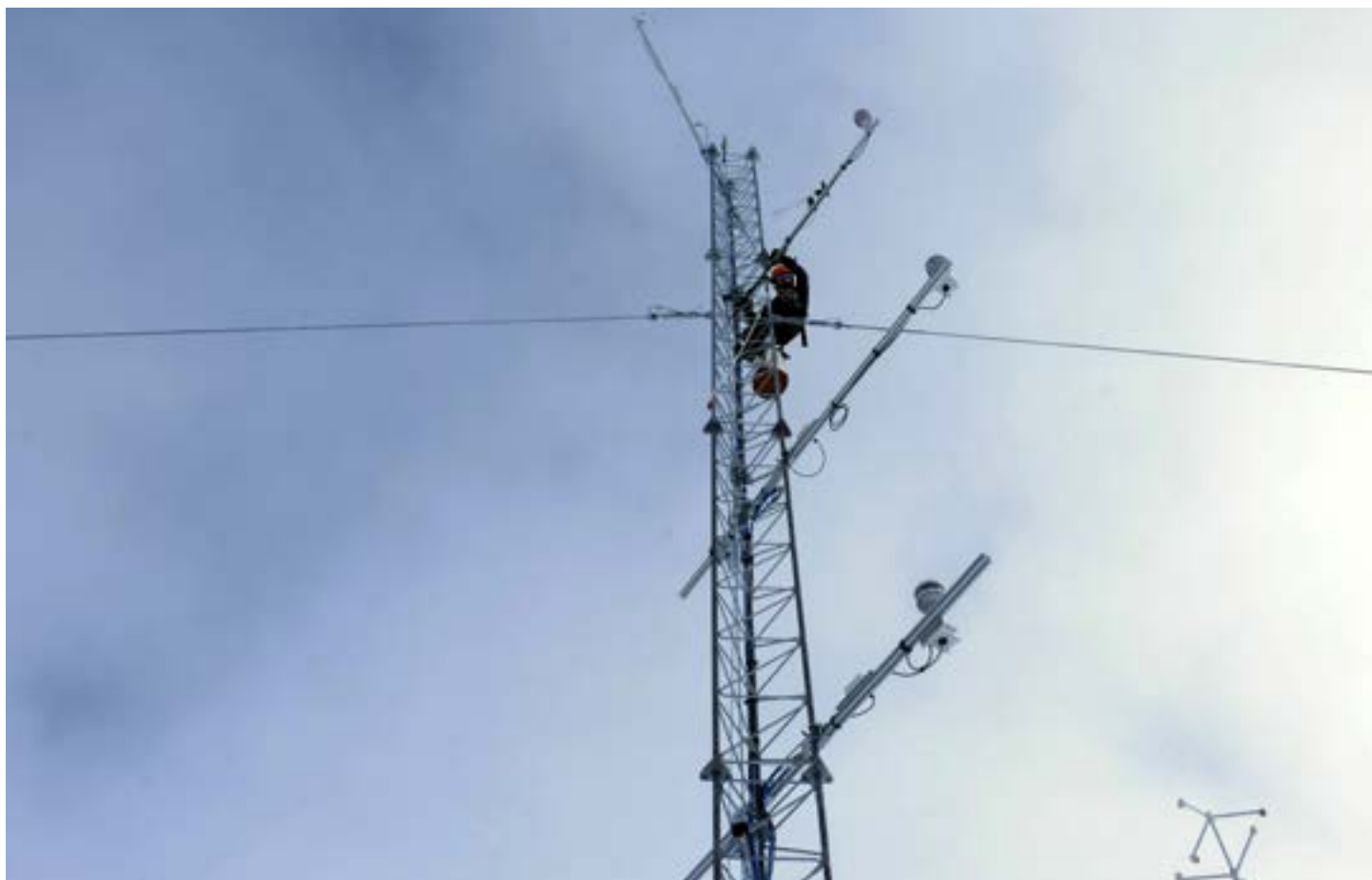
A CIESRDS researcher climbs a tower at Summit, Greenland, to install and align an anemometer as part of the NOAA Federated Aerosol Network (NFAN).
